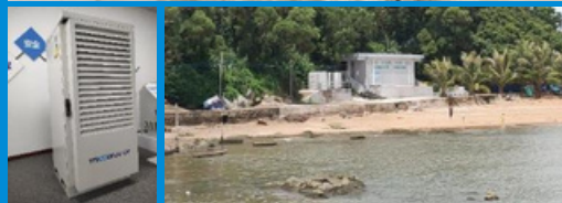
Backup power source for telecom services Demonstration unit in Mangzhou Island--5G Hydrogen Energy Smart Island
